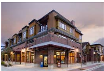
◀ City of Dallas 2-story mix, residential over commercial
